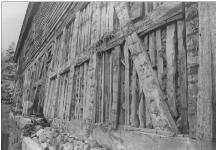
Lutze house barn, c. 1847, Saxon German, near Cleveland. Note half-timber construction.
