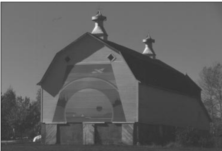
Gambrel roof, one of the most popular roof styles found in Wisconsin, near Washburn.
