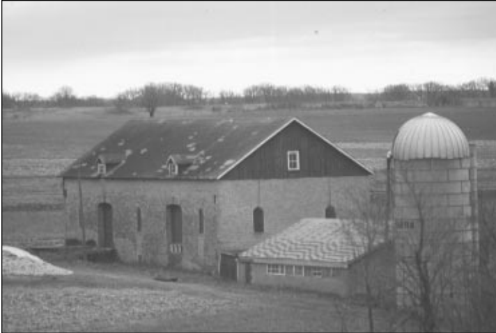
Occasionally, the entire barn was constructed of quarried rock.
