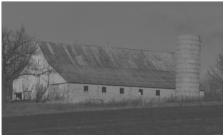
Gable roof with a lean-to on each side, east of Mineral Point.
