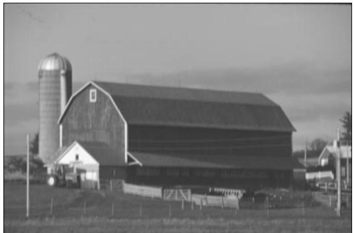
Swiss barn near New Glarus. Note pentroof above the windows.
