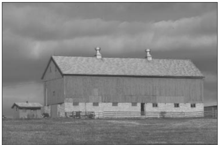
Several styles of roofs were used in building Wisconsin's historic barns. An early style used was gable, south of Spring Green.
