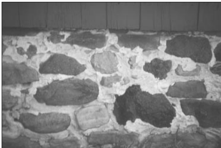
Where field stones were readily available, they were used.
